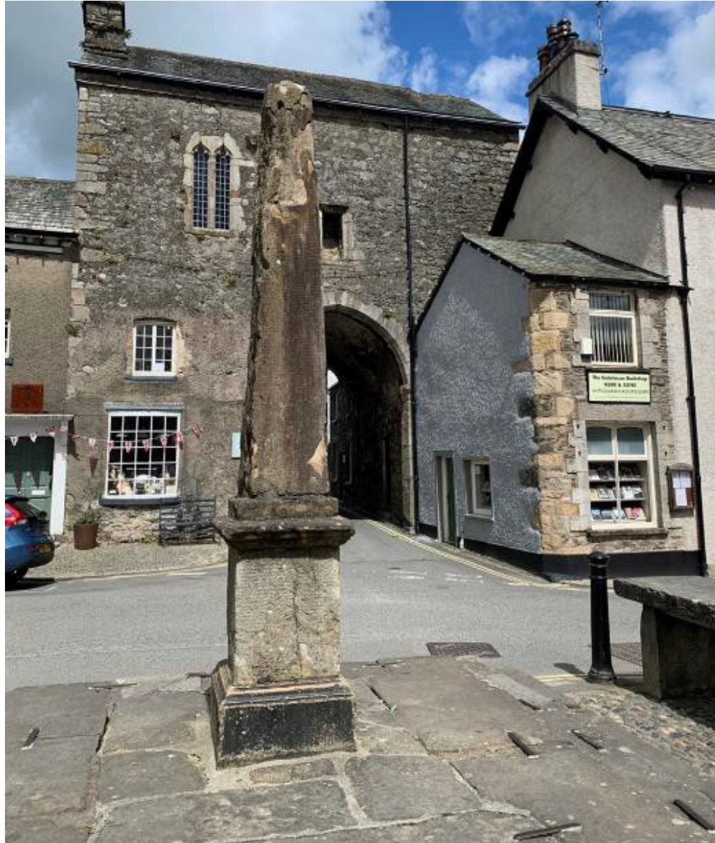
Figure 30: Historic surfacing in Cartmel includes sandstone flags and cobbles, which should be retained.
